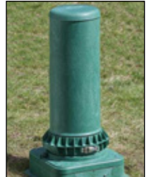
Installed 28" GLC with Grounding Spacer
