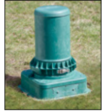
Installed 17" GLC with Grounding Spacer
